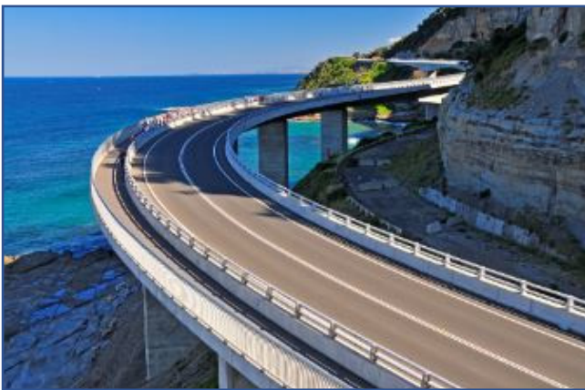
Picture: Sea Cliff Bridge | NSW
